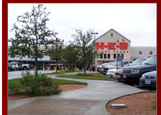
On-site pedestrian ways are an important part of site design (shown: grocery store).
