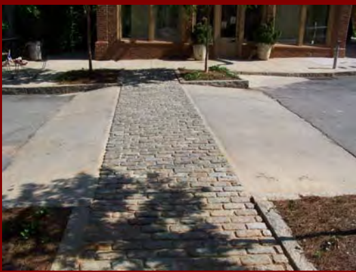
Speed tables may be used effectively to "calm" traffic while also serving as an amenity.
