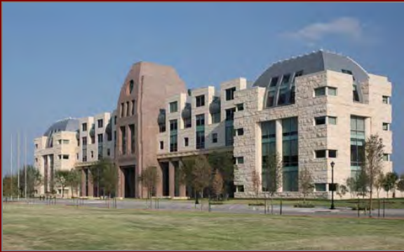
The City of Frisco, Texas recently built a joint City Hall and Library that features green design concepts.
